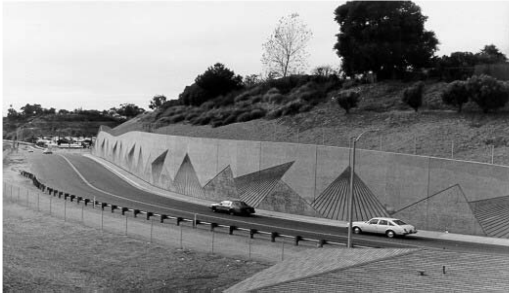
Figure 4.11: Cast-in-Place Facing.
