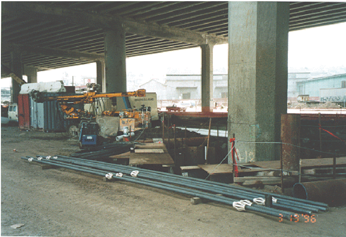
Figure 8-3. Storage of Reinforcing Steel.
