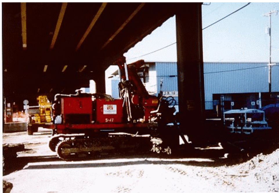
Figure 3-6. Underpinning of West Emerson Street Viaduct, Seattle, Washington.
